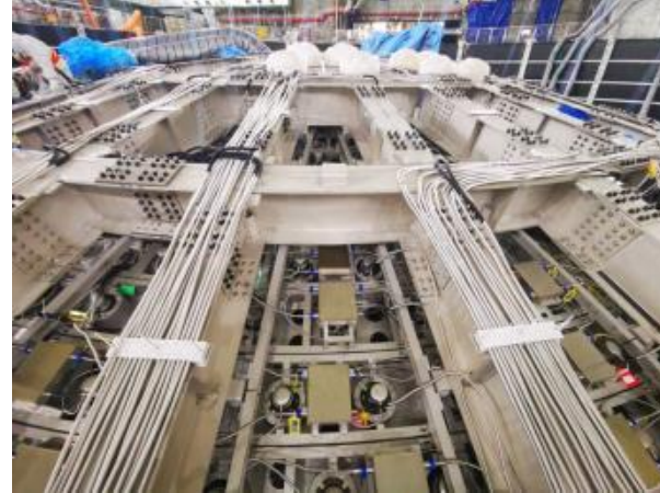
Installation on the steel structure
