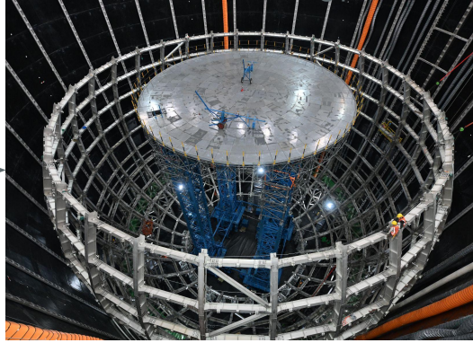
Acrylic vessel installation until equator
