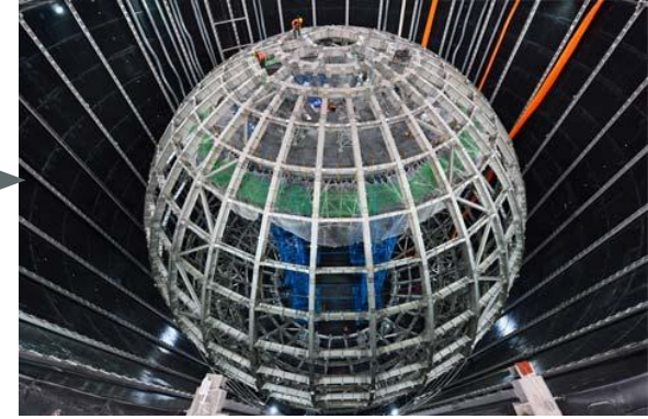
Acrylic vessel completed
