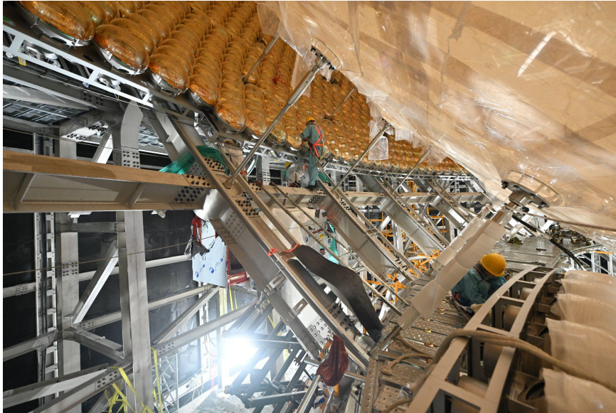
Installing the PMTs after acrylic panels
