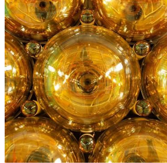
Installed LPMTs and sPMTs
