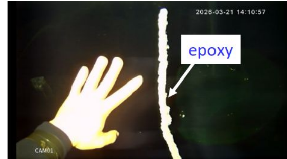
2nd crack with epoxy and divers hand
