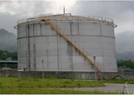
5000 m 3 tank LAB tank
