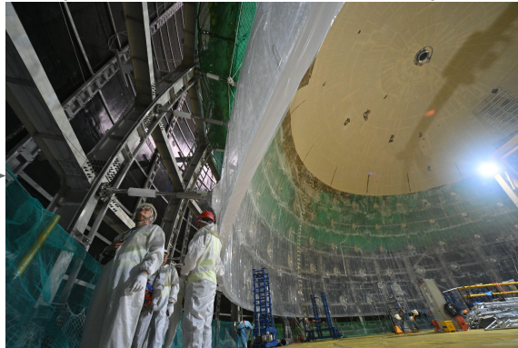
Acrylic vessel installation until equator
