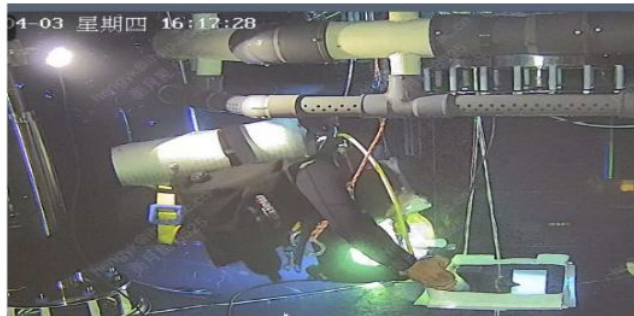
Diver applying glue to close the first crack,
