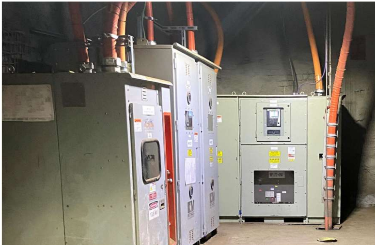
Remote operated breakers
