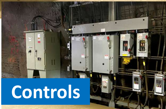
Remote operated breakers
