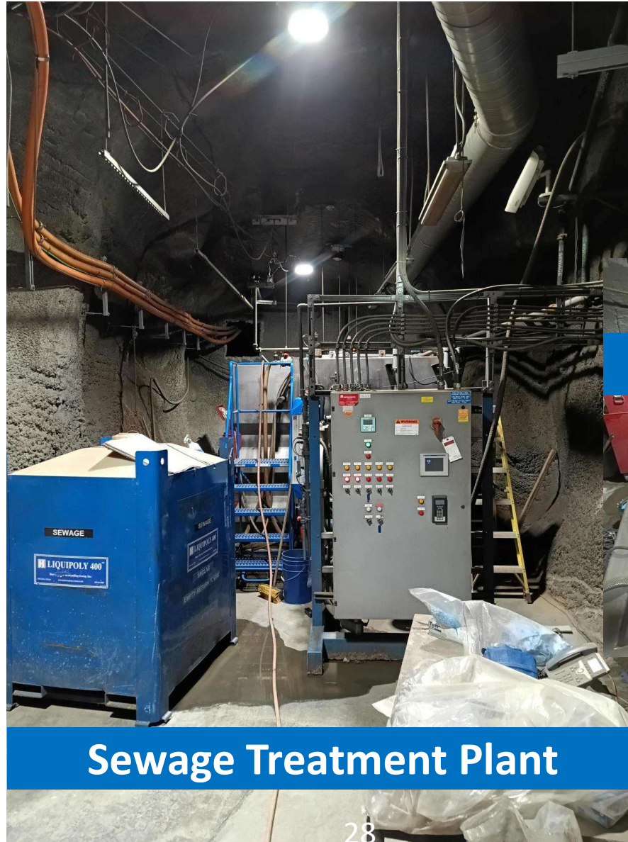
Membrane Bio-reactor
