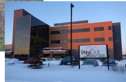
SNOLAB Surface Building
