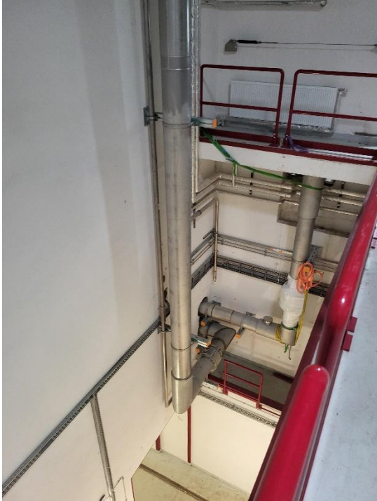
Cryo-lines installed in „Shaft east“
