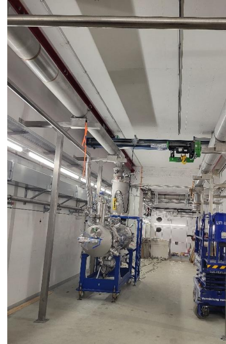
Cryomodule 2 connected to cryo-line in „beam position“ at corridor East
