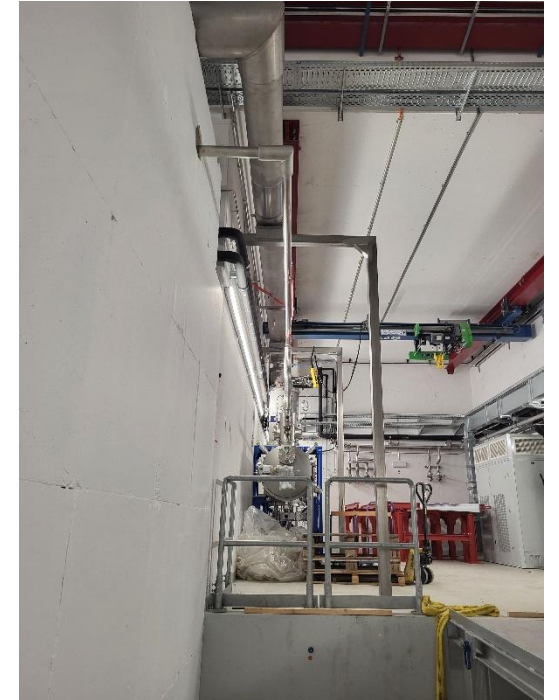
Cryomodule 1 connected to cryo-line in „beam position“ at corridor West
